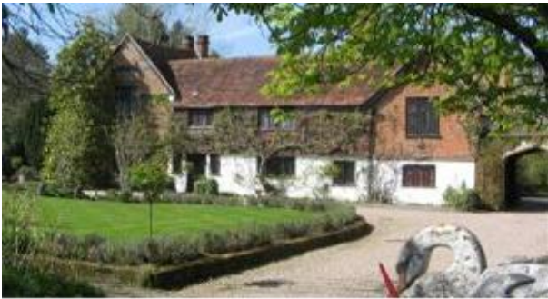
Lucas Green Road Heritage Asset - Lucas Green Manor and Barn, Grade II listed.
