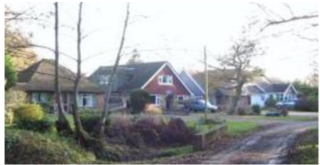
Priest Lane A row of chalet and single storey bungalows built in the 1930s and 1960s.
